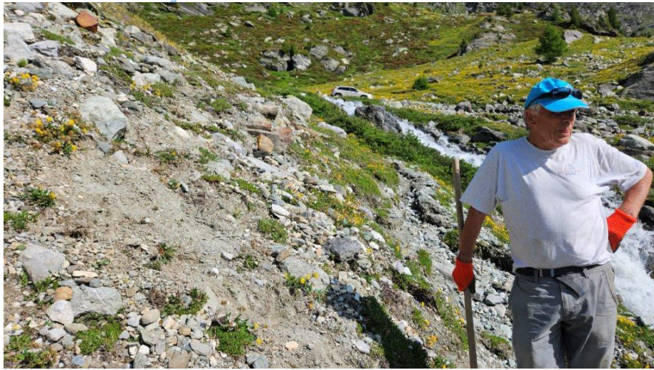
Demolish path before
